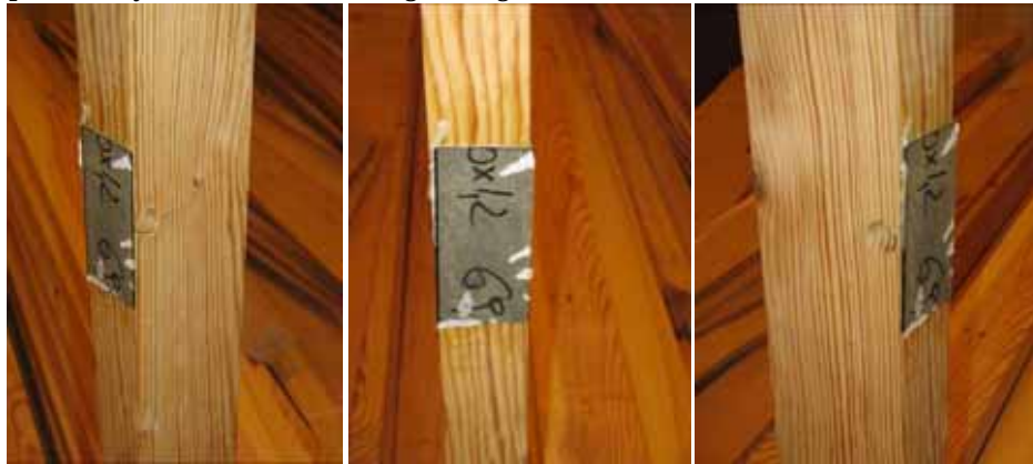
Figure 3. Timber beams locally reinforced with CFRP tape
